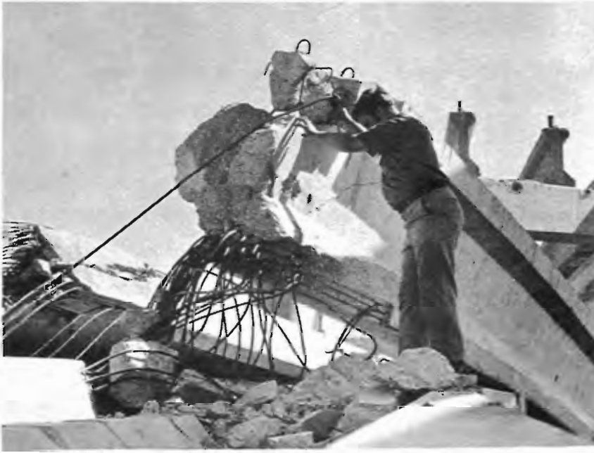
Fig. 2. Sections of 109,000 lb. beams at U. S. 82 and Parkway Drive interchange which were blown down by the first tornado. (Courtesy of Mr. Milton Adams, Lubbock Avalanche Journal photographer)
