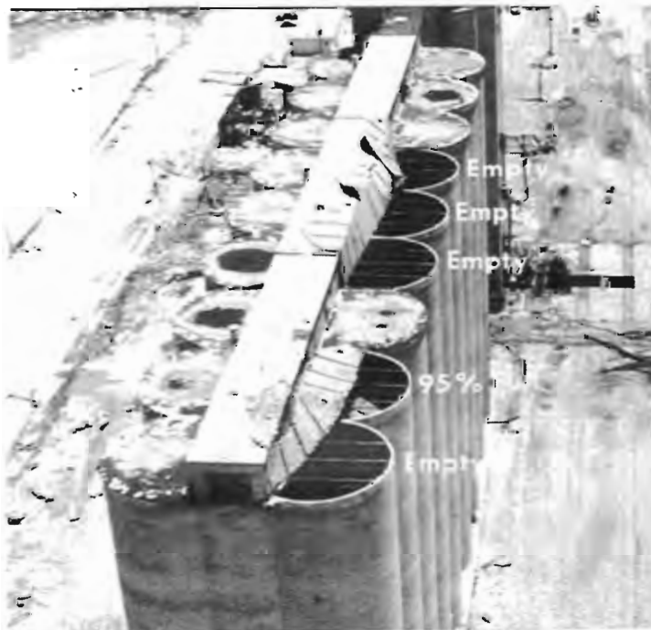
Fig. 15. Lifted tops of grain storage bins at Goodpasture, Inc. Tops were made of 10-inch thick concrete and had a diameter of 33 feet. Note that the second one was 95% filled with grain while others damaged ones were empty.
